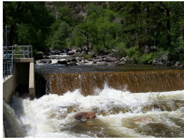
Our diversion dam in Big Goose Canyon
